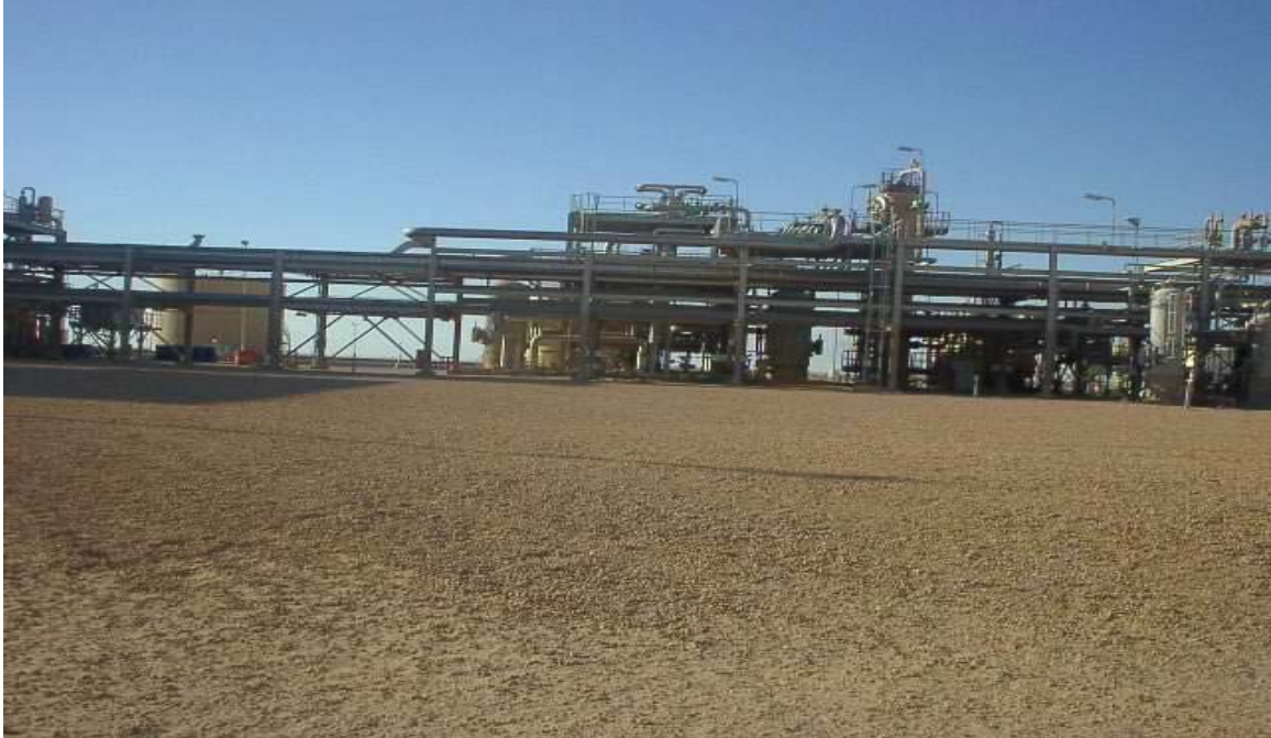
Salam Gas Plant (Khalda)
