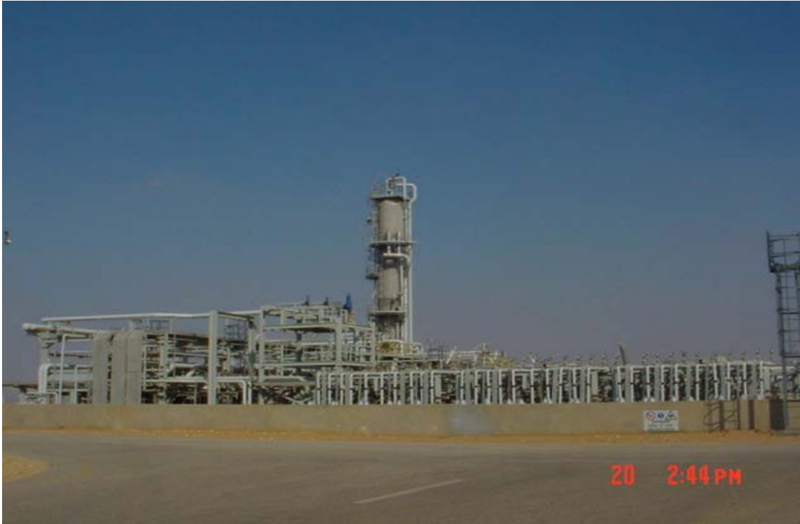
Qarun Oil Process Facility
