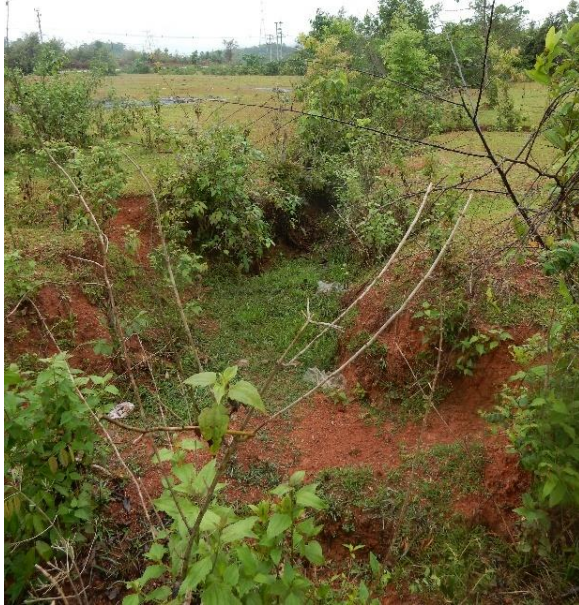
Plate 4-1 Drainage channel, Mill footprint
