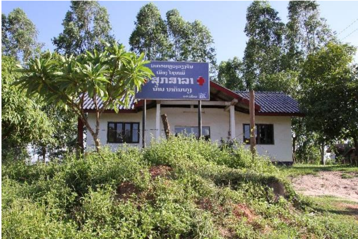
Plate 6-19 Health Centre in Ban Nakhathoung
