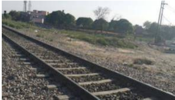
Crossing Station P7 (parallel)/New Khatauli
