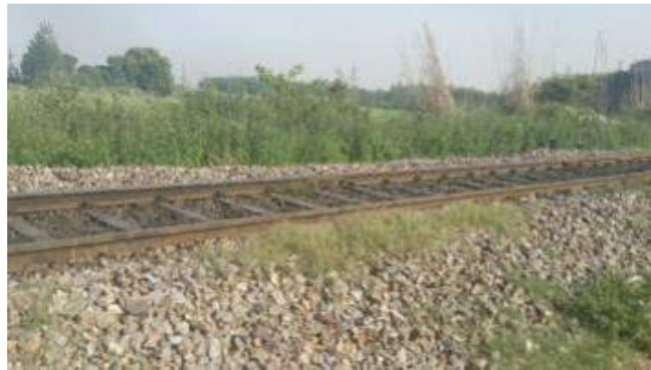
Crossing Station P6 & IMSD (parallel)/New Sakoti
