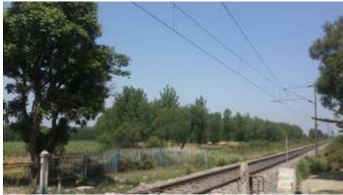
Crossing Station P9 (parallel)/New Talheri Bujurg
