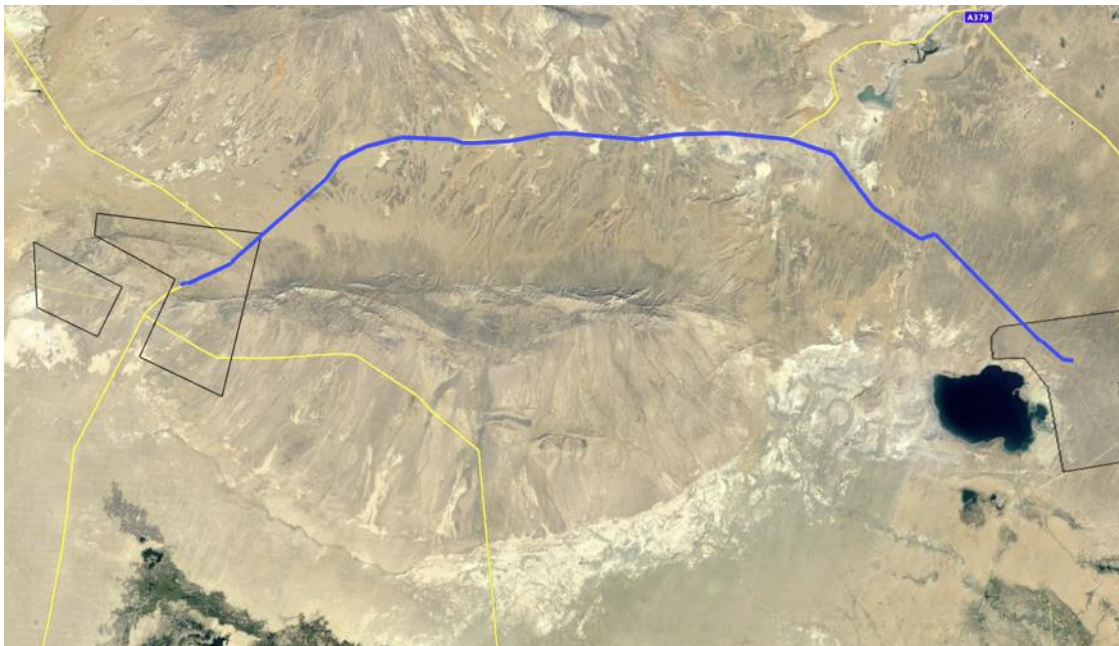
Figure 4-8 Route of Transmission Line Mostly Through Desert Land
