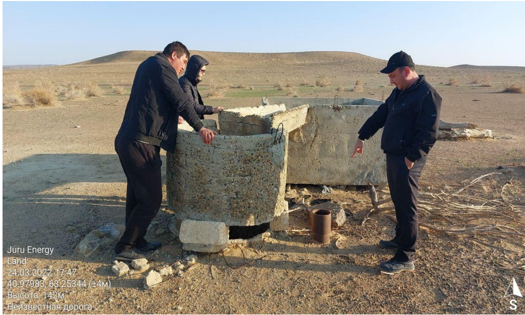
Ataniyaz Well 2 – Can be used by herder 2 upon renovations
