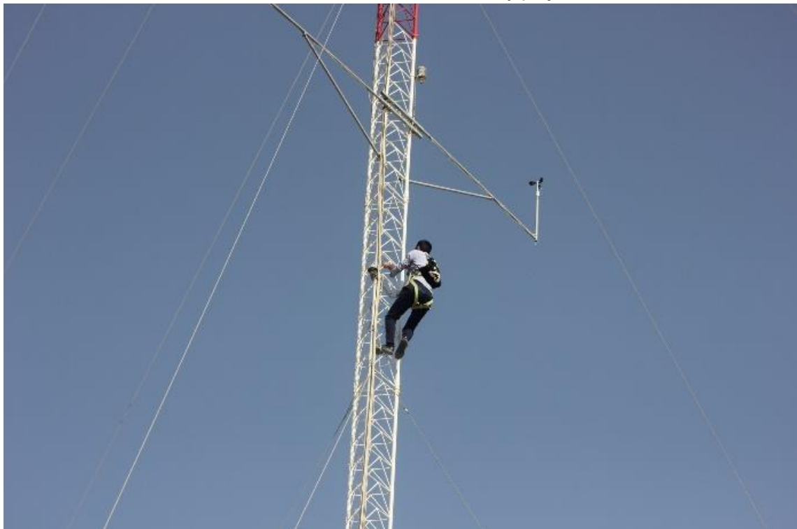
Bat detector installation on weather mast in Dzhankeldy project area
