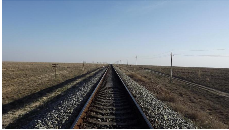
Plate 2-7 Railway Line crossing the Project site
