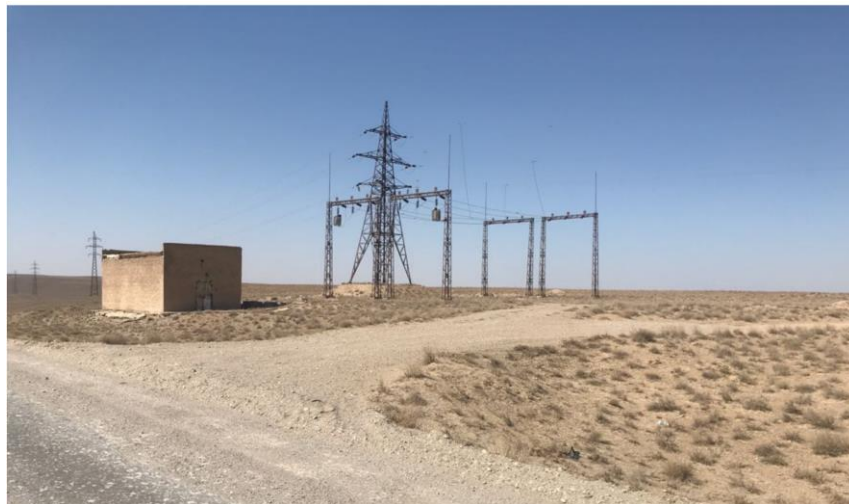
#R31– View of the OHTL and structure owned by grid operator
