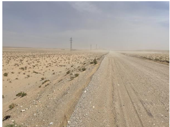
View of the OHTL along the Access Road
