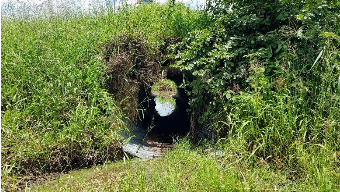
Culvert 1: 673255.68 m E , 8402690.36 m S
