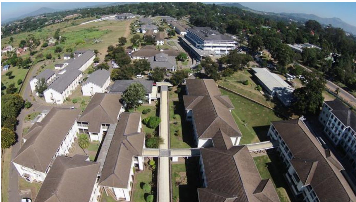
Figure 1.1 An overview of picture of the College of Medicine Campus in Blantyre
