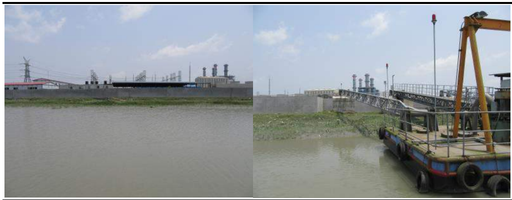
Figure 0.11 Existing Bhola I Premises
