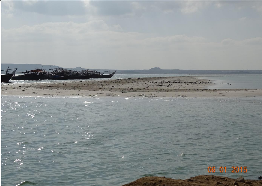
Figure 6-17: View to the South of root of LBW (Photograph taken on 6-Jan-2015)
