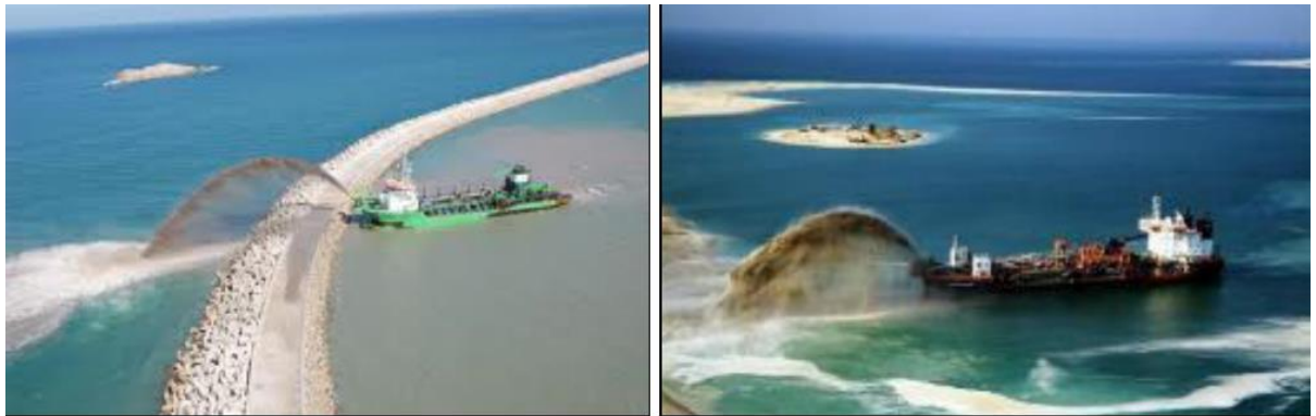
Figure 3-11: Examples of Rainbowing by Dredgers
