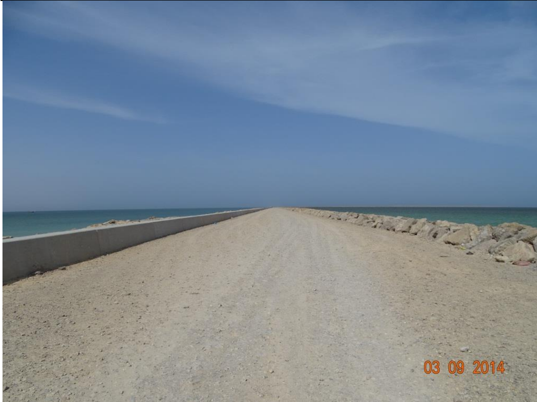
Figure 6-16: Photograph of the Existing LBW (Photograph on 3-Sep-2014)
