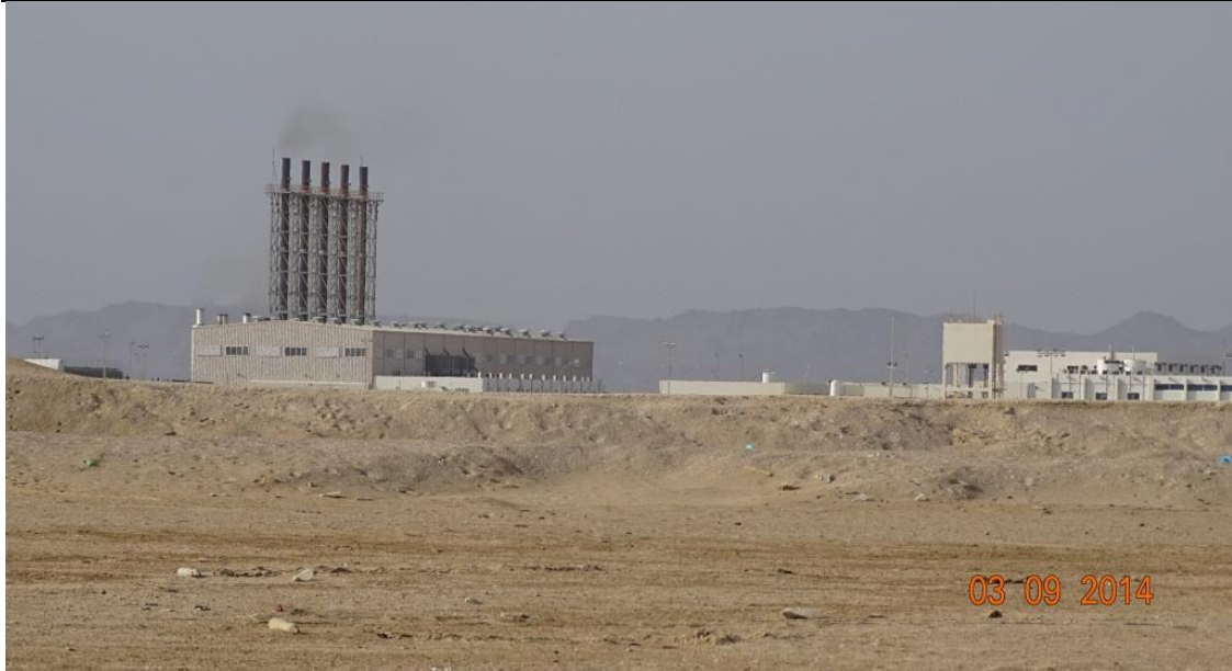
Figure 3-14: Existing Power Plant in Duqm (Photograph 3-Sep-2014)
