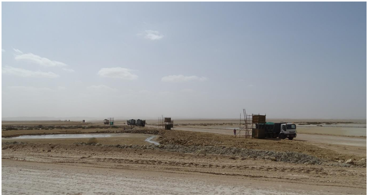
Figure 6-15: Truck Movement near the LBW (Photograph on 20-Aug-2015)
