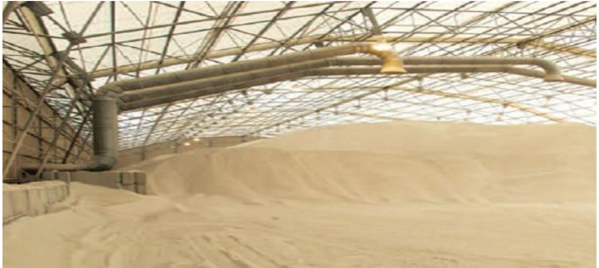
Figure 3-3: Example of a Steel Frame Fabric Storage Building
