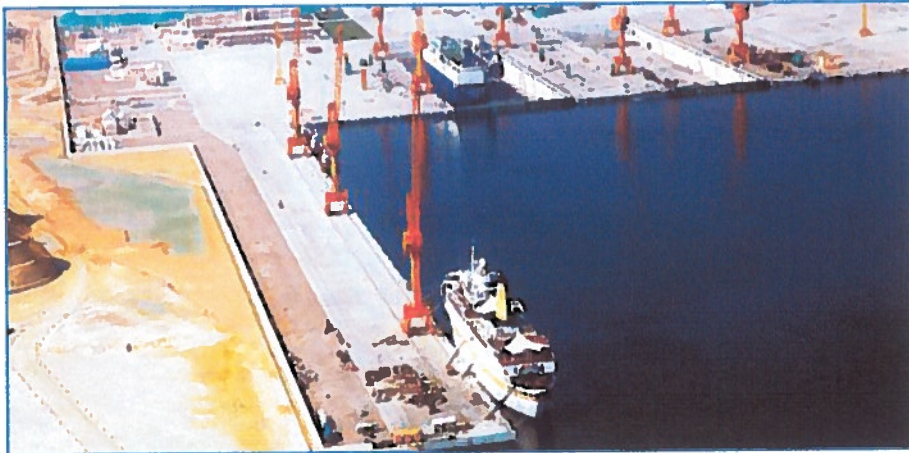
Figure (6. 8 ) : Surrounding environment, Dry Dock facility impacting on the proposed packages, (Photo taken by SEZAD)
