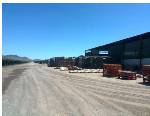
Photo 4. Typical Store- and Pack House Complex
