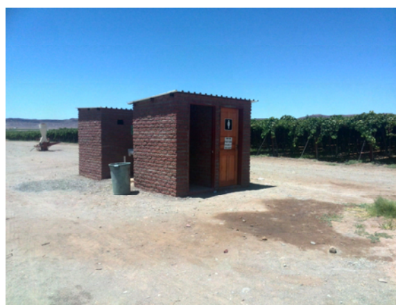
Photo 3. Typical VIP Toilet Amongst Vineyards
