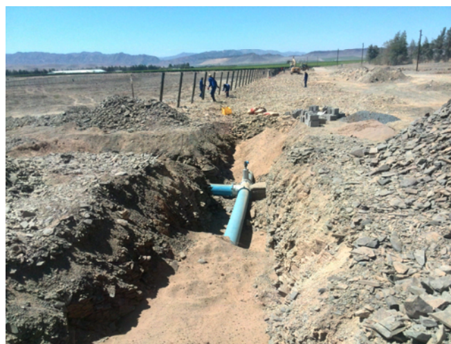
Photo 2. Typical Construction of Drainage system
