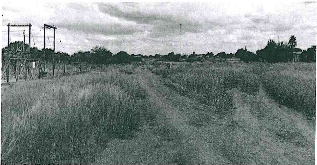
Figure 4: The installation site for the proposed renewable PV solar power plant in Gobabis.
