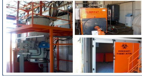
Photo 2: View from inside the facility
