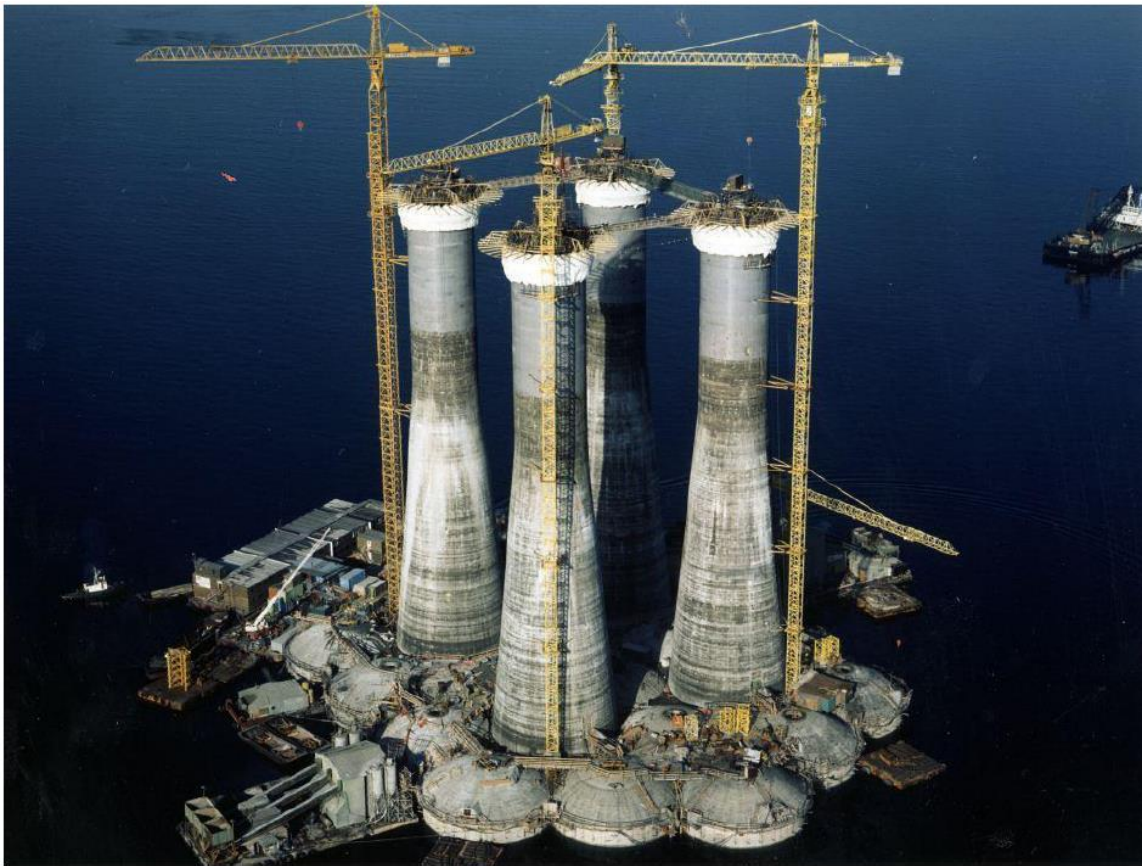
Photograph 3.0-3: Concrete construction with liquid storage tanks in Norway
