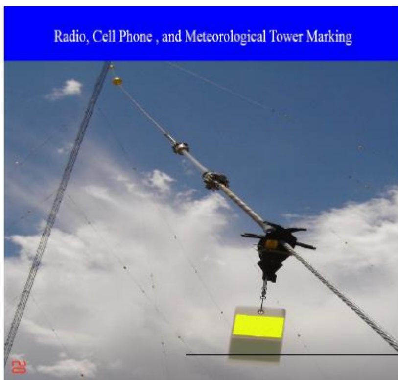
Photograph 4.9.1: Reflector for marking cables 41
