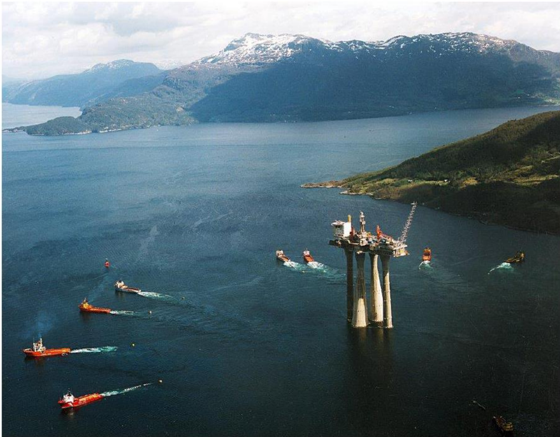
Photograph 3.0-2: Transportation of a gas treatment facility on a concrete construction to the offshore treatment site in Norway
