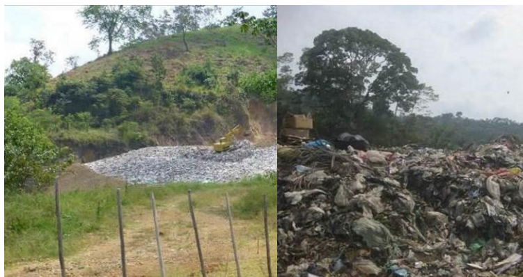
Controlled dump in El Progreso
