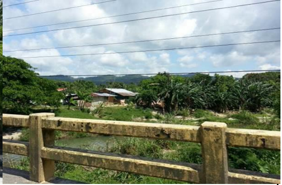
Bridge over La Esperanza River
