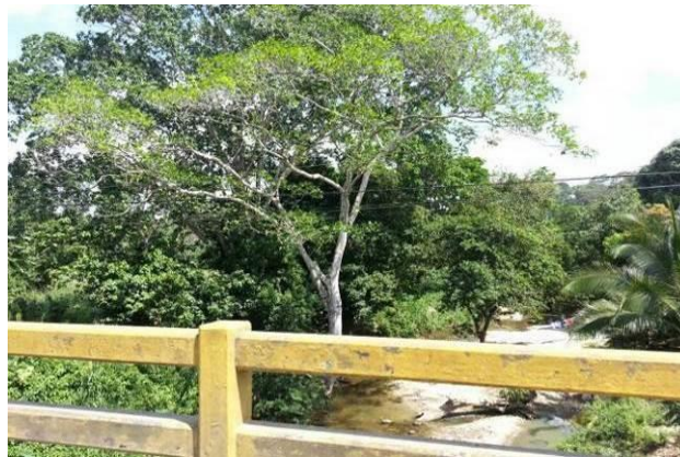
Highland Creek Bridge
