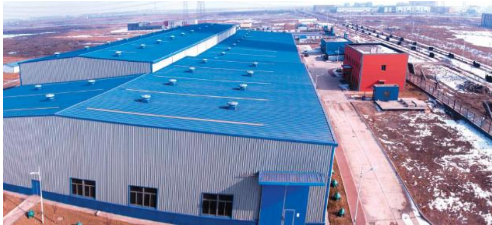
Figure 5 Example of Project Site layout, photo of Caofiedian desalination facility building structures with a similar layout to the proposed Project
